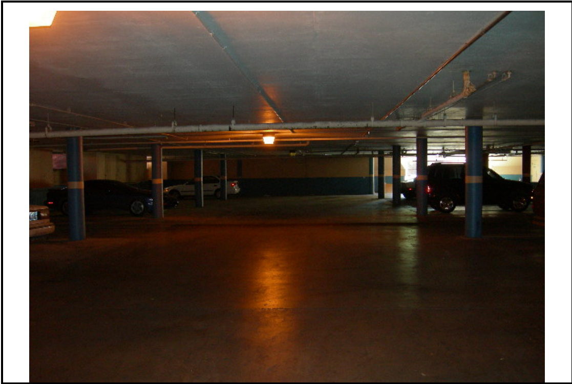
Underground parking garage
