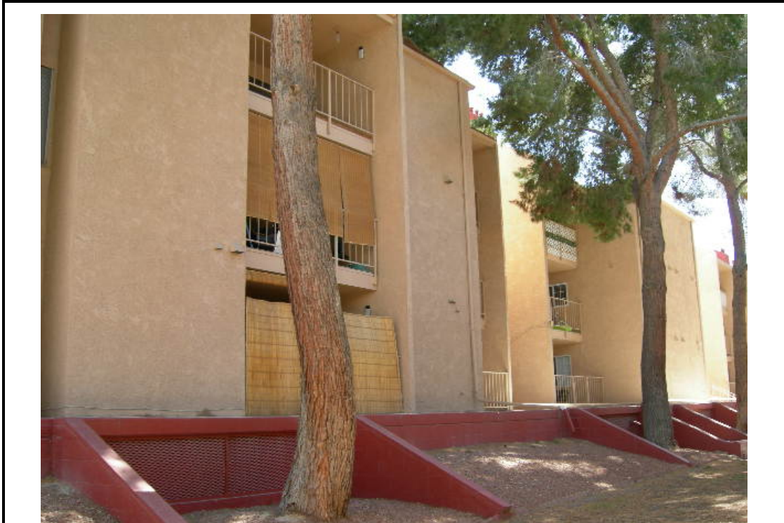
View looking west at the subject's 3-story building
